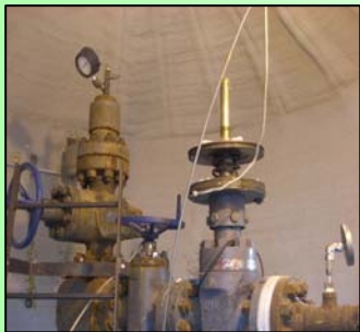
SSV actuator (minus the housing)
